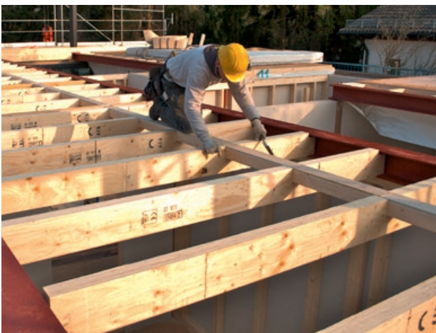
STEICO LVL R used for the construction of high load bearing floor structures
